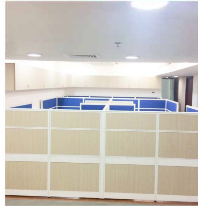
Location: Gurugram (Haryana) Date: 2016 Client: Fortum India Pvt Ltd Type: Corporate Office (Renovation) Build up area
